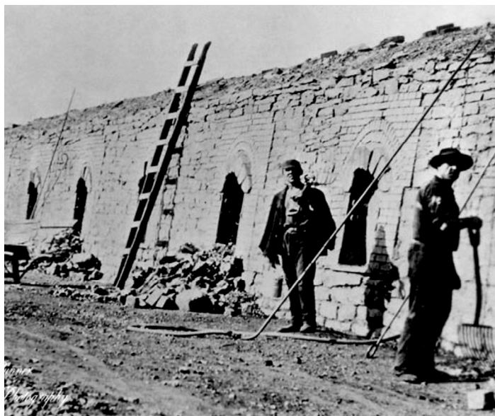
Figure 25. Beehive coke ovens operated in Star Junction. The coke ovens were in Stickel Hollow on the Washington Run Railroad, which later was owned by the P&LE Railroad. It appears that the rail bed became the four-lane PA 51 (from Boyles, 2018).
