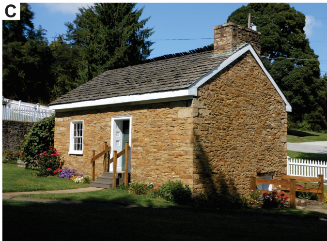
Figure 56. A – The Abraham Overholt Homestead, built in 1838, is now the headquarters of the West Overton Village & Museum. B – The Overholt Distillery, built in 1859, also housed a steam-powered grist mill. The building is now the museum for West Overton Village & Museum. C – This springhouse associated with the Abraham Overholt Homestead is where Henry Clay Frick was born.
