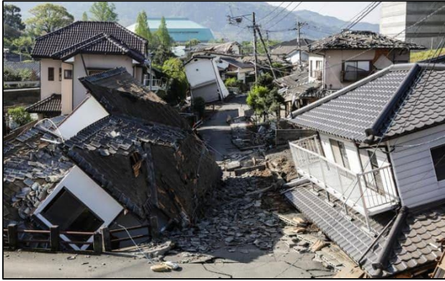
Some of the devastation from the 2016 Kumamoto earthquake
